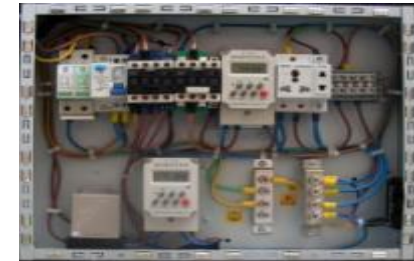
AC electrical control module
