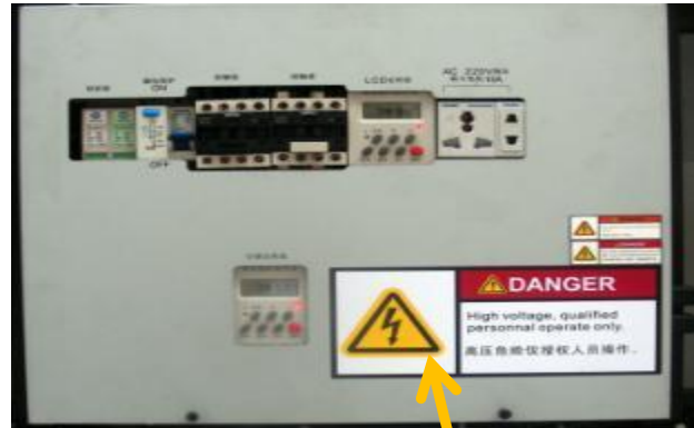
AC power control module
